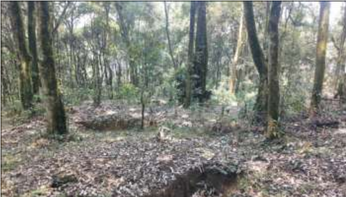
Recharge structures in the 40 acre forest land of Tendong hills. The forest landscape approach springshed revival works.
