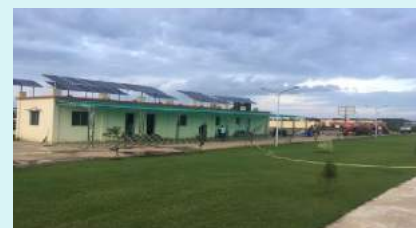
Solar power plant at Bhubaneshwar FSTP
