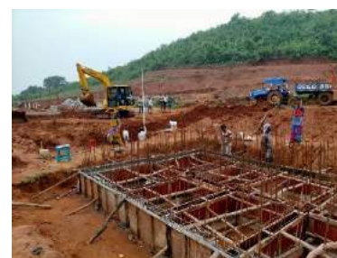
Figure 9: A plant under construction in Odisha
