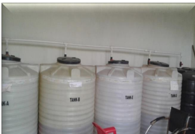
Different fertilizer tanks fitter with micro irrigation system unit Abohar Punjab
