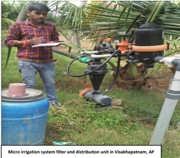
Micro irrigation system fitted with opens well in Visakhapatnam, AP
