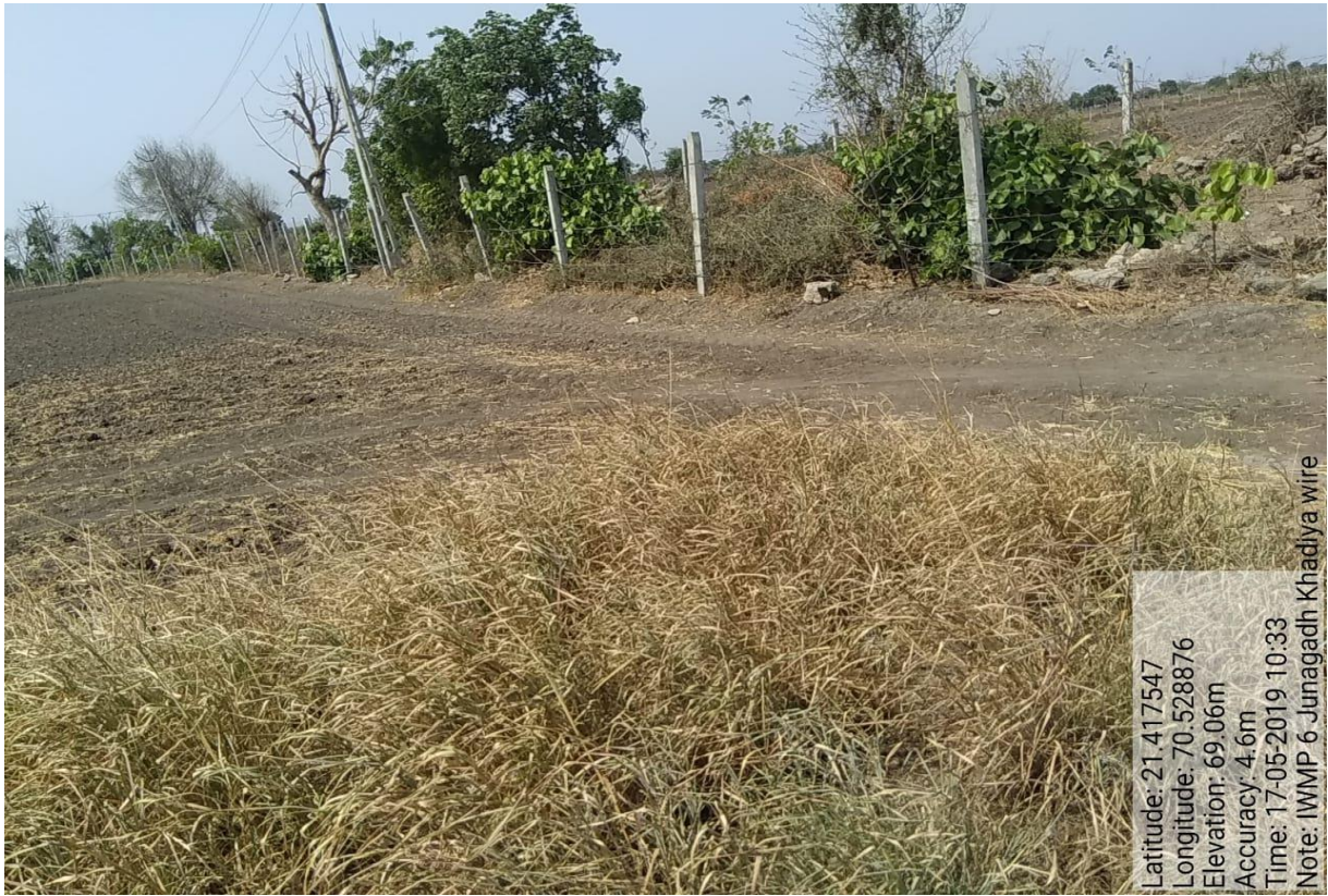
WAPCOS TEAM VISITED FIELD WIRE FENCING WORK IN IWMP-VI JUNAGADH
