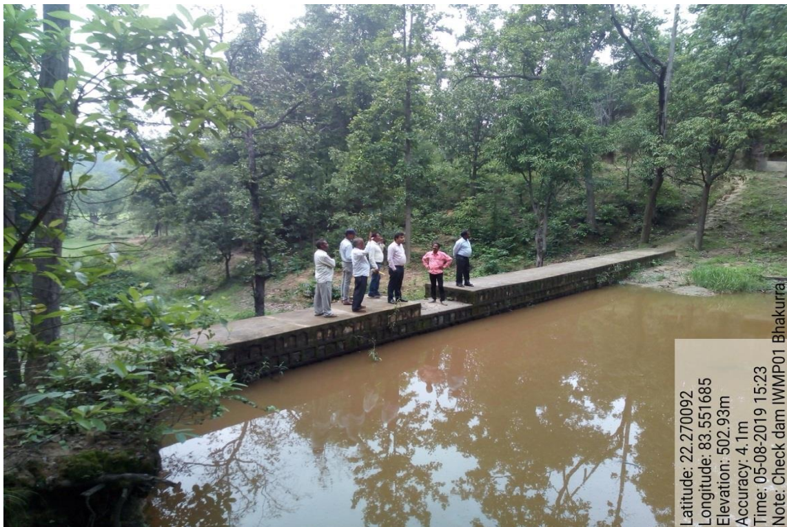
WAPCOS TEAM VISIT CHECK DAM IN IWMP-I RAIGARH
