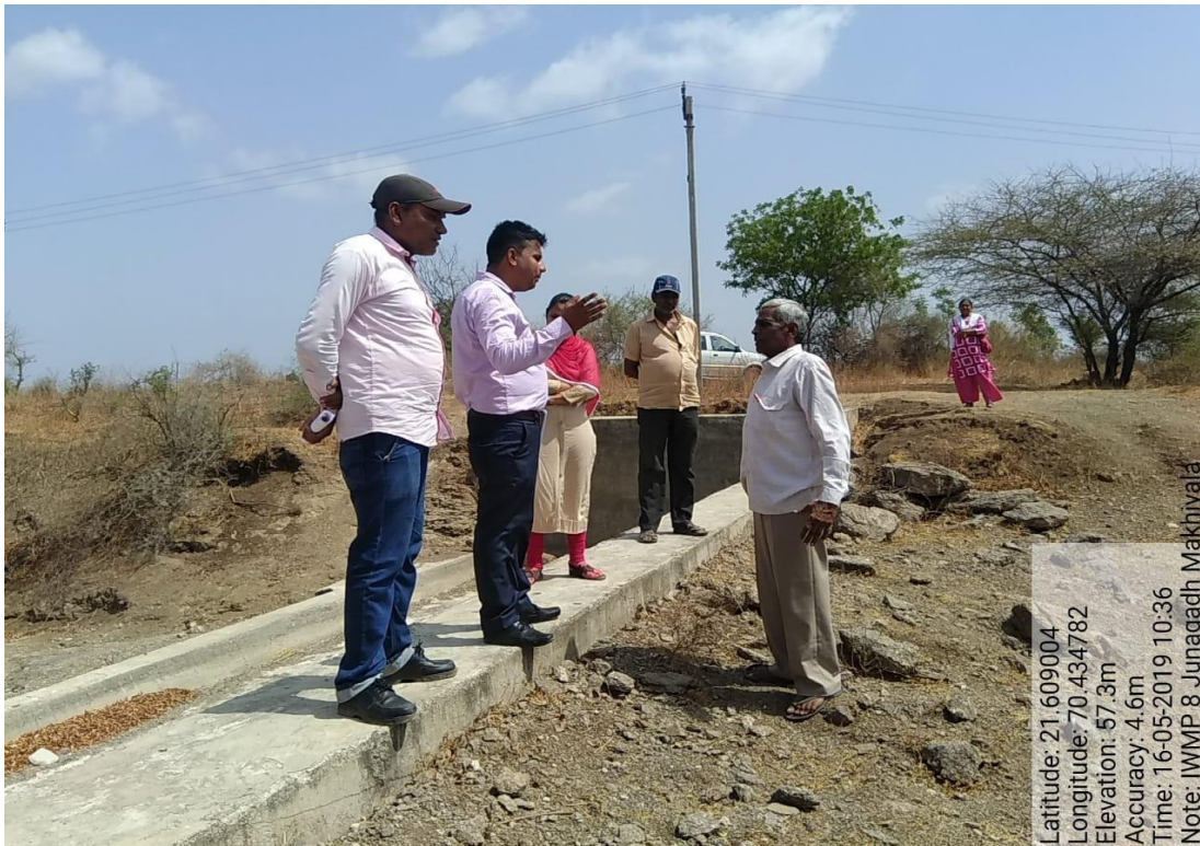
WAPCOS TEAM VISIT CHECK DAM IN IWMP-VIII JUNAGADH
