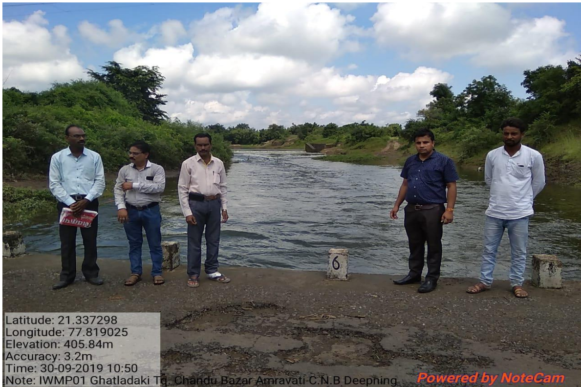
WAPCOS Experts Discuss with Officials and Visited the Water Harvesting Structure of IWMP-I
