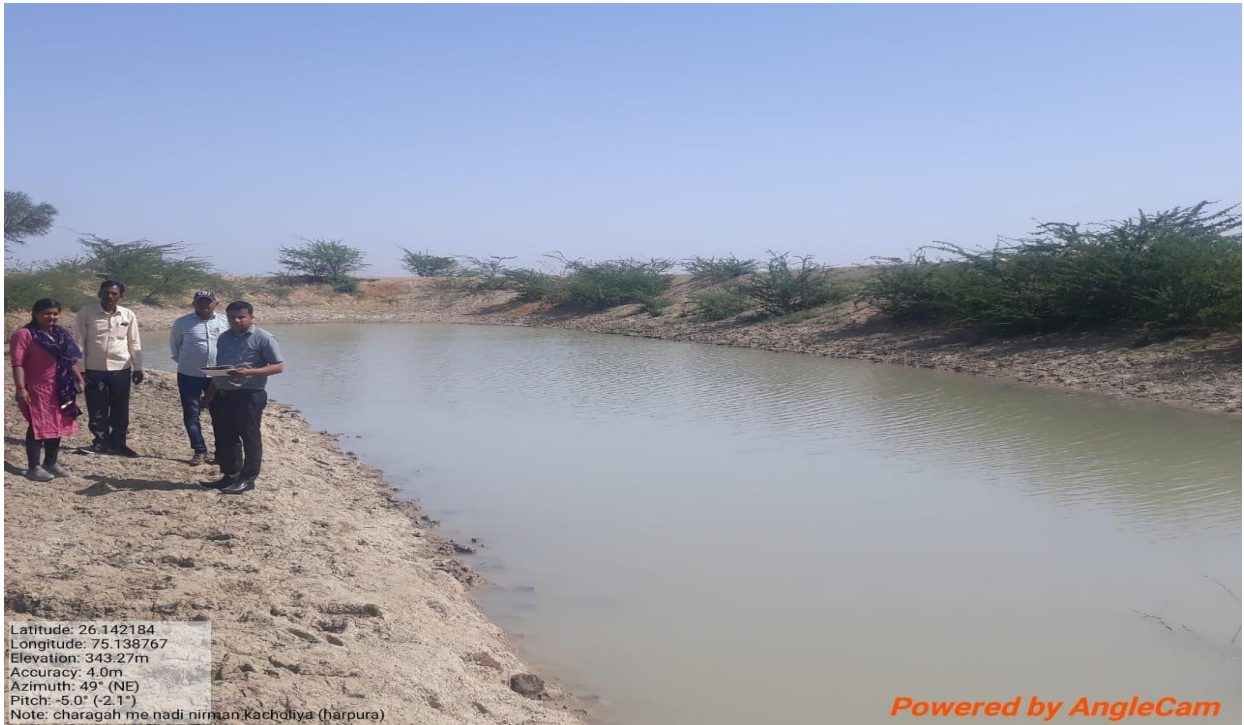
CONSTRUCTION OF NADI IN CHARAGAH VILLAGE KACHOLIYA IWMP-V ARAIN AJMER
