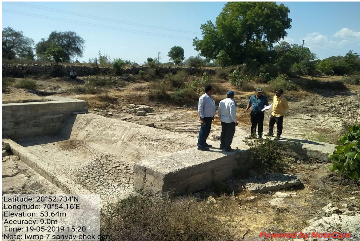
WAPCOS TEAM VISIT CHECK DAM IN IWMP-VII JUNAGADH
