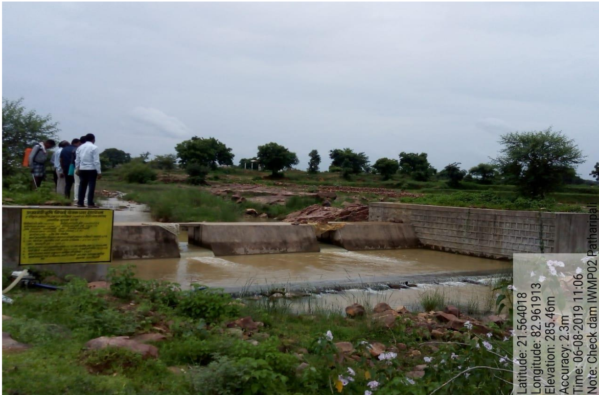
WAPCOS TEAM VISIT CHECK DAM IN IWMP-II RAIGARH
