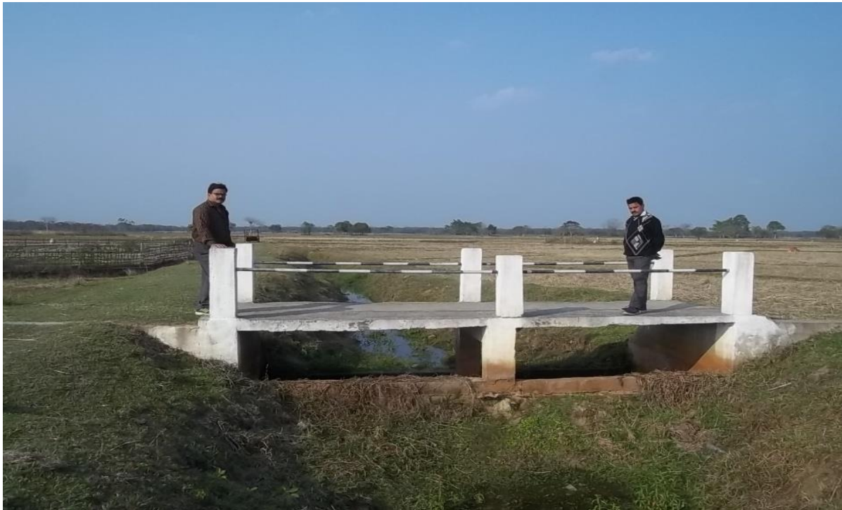
WAPCOS EXPERT VISIT RCC CHECK DAM IWMP-1 BLOCK MATIA GOALPARA
