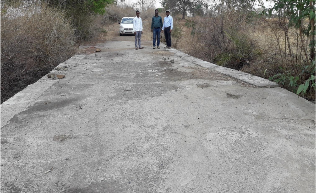
WAPCOS TEAM VISIT CAUSE WAY CUM CHECK DAM IN IWMP-I BHOPAL
