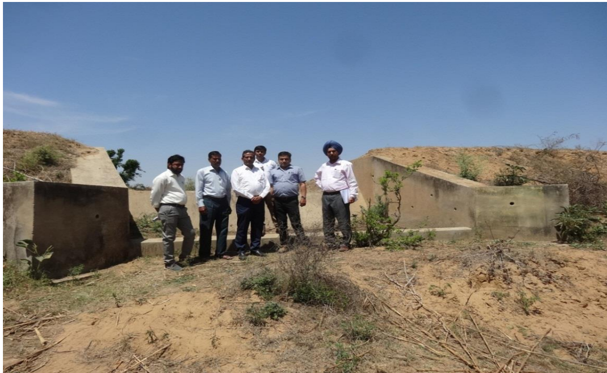
WAPCOS EXPERT VISIT CHECK DAM IN DISTRICT ALWAR
