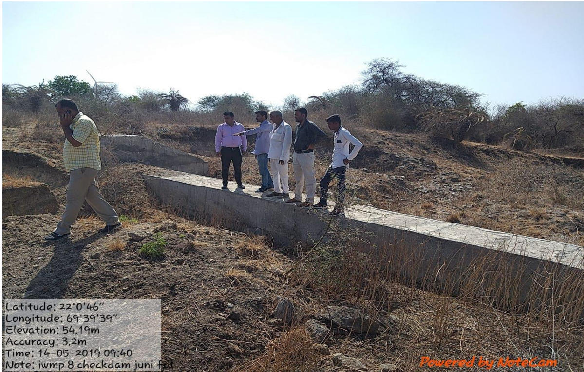
WAPCOS TEAM VISIT CHECK DAM IN IWMP-8 JAMNAGAR GUJARAT
