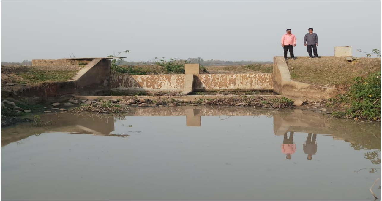
WAPCOS EXPERTS VISIT RCC CHECK DAM IWMP-II GOALPARAJ AYRAMKUCHI
