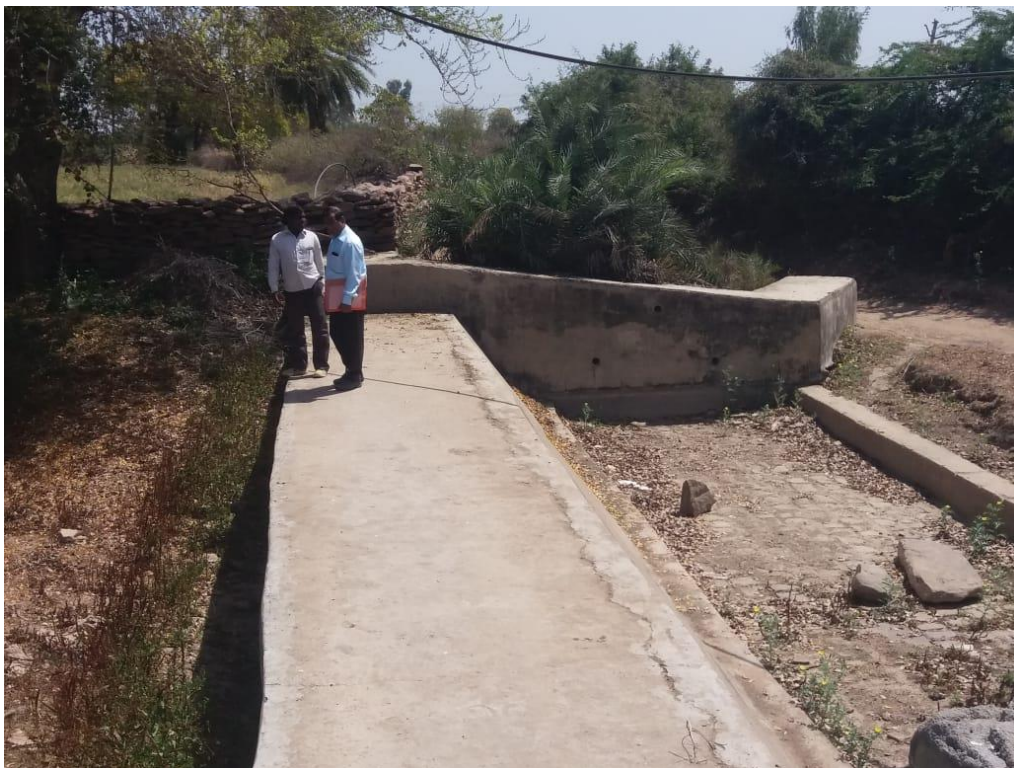
APCOS OFFICIALS VISIT CHECK DAM IN IWMP-VII BANASKANTHA
