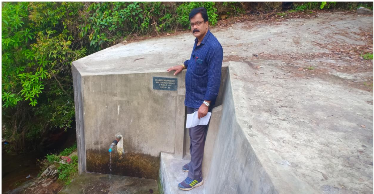
WAPCOS EXPERT VISIT STORAGE TANK WORK IN IWMP-IV BLOCK MYLLEIN MEGHALYA
