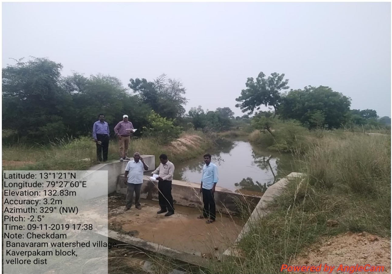
WAPCOS Experts Discuss with Officials and Visited the Water Harvesting Structure of IWMP- II, Kaveripakkam
