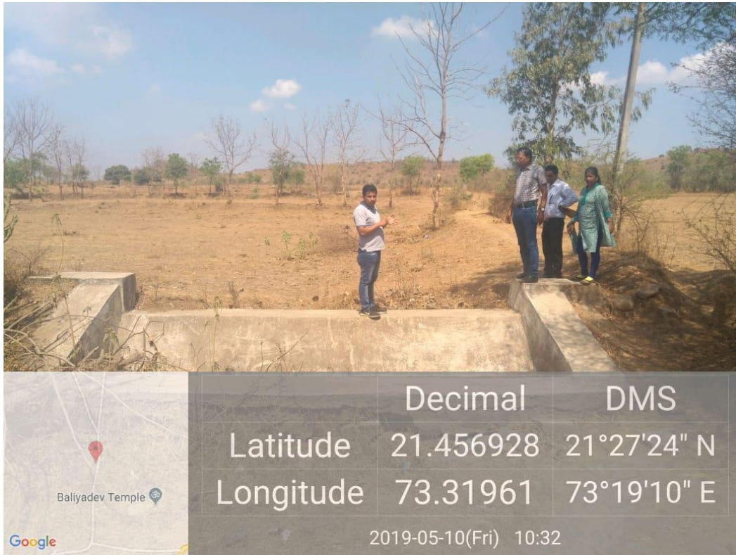
WAPCOS TEAM VISIT WASTE WEIR AT IWMP-I VAD SURAT GUJARAT
