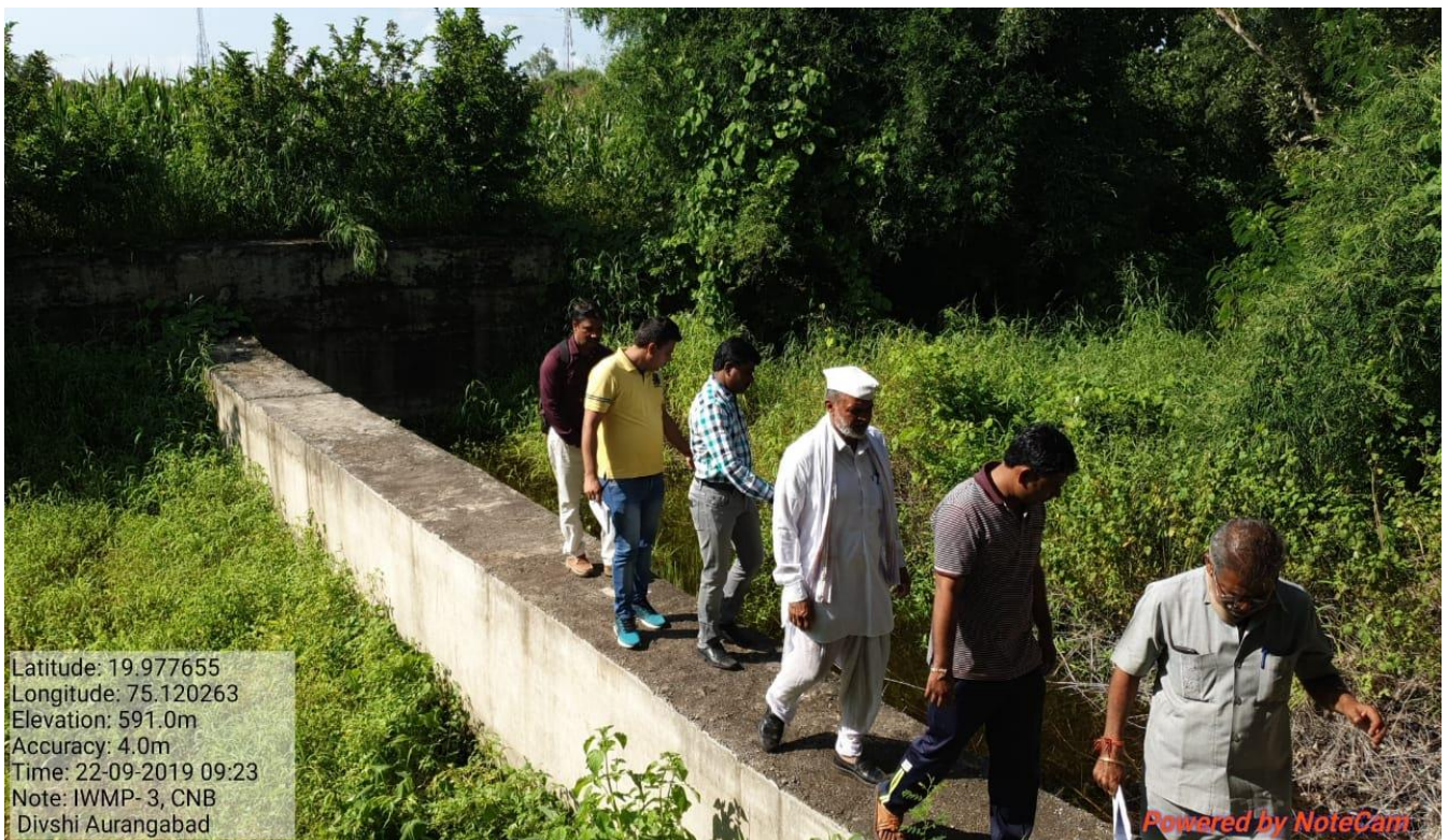
WAPCOS Experts Visited the Micro Irrigation System & Check Dam of IWMP-II
